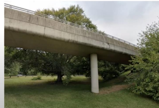
Existing MVT bridge crossing
