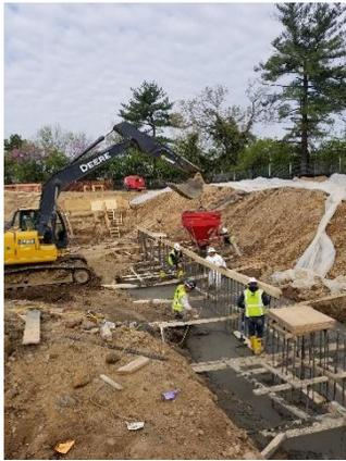
1500 geo-piers were placed in the ground to support the building and contaminated materials were excavated and placed in their secure locations. Over the last several weeks – we now have a pool!.....sort of.
